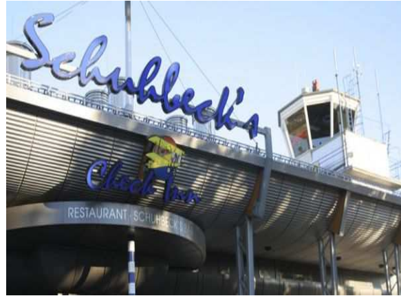
Restaurant Schuhbeck's Check Inn Flugplatz Egelsbach
